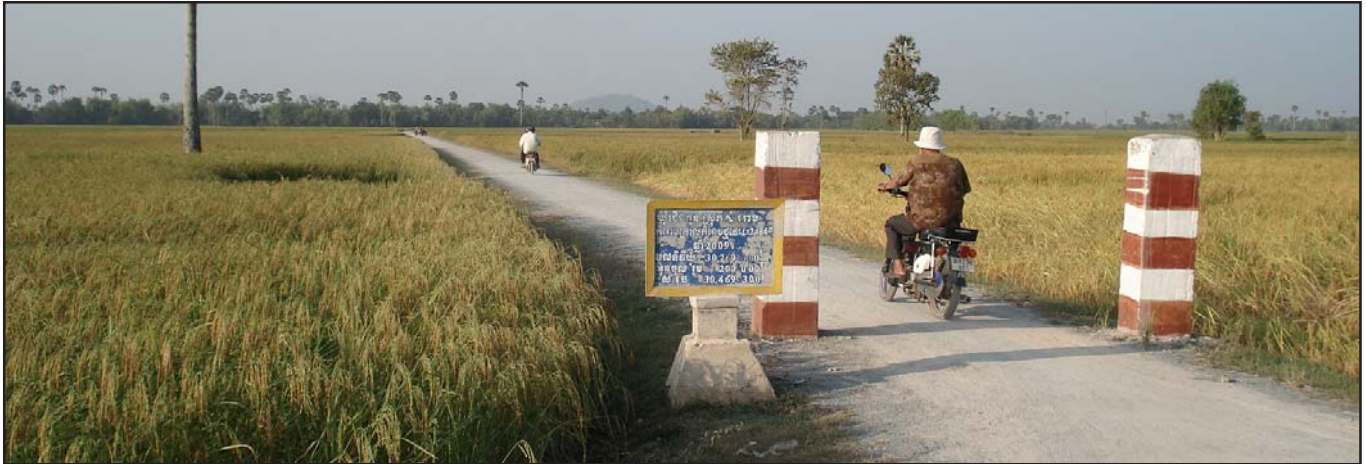
This 2.1 km commune road was built in Cheung Koun Commune of Samrong District, Takeo Province, in 2009.
